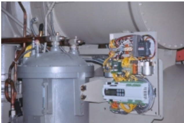
Figure 2, Compressor Controller
