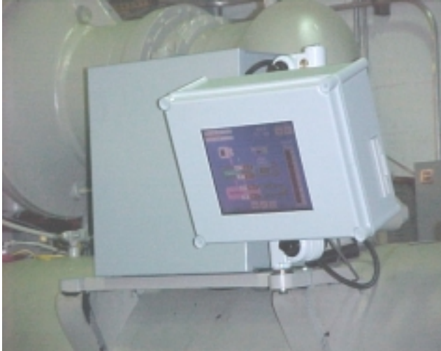
Figure 1, Unit Controller and Operator Interface Touch Screen
